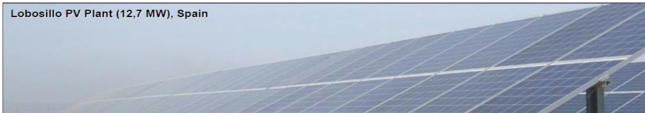
Lobosillo PV Plant (12,7 MW), Spain
